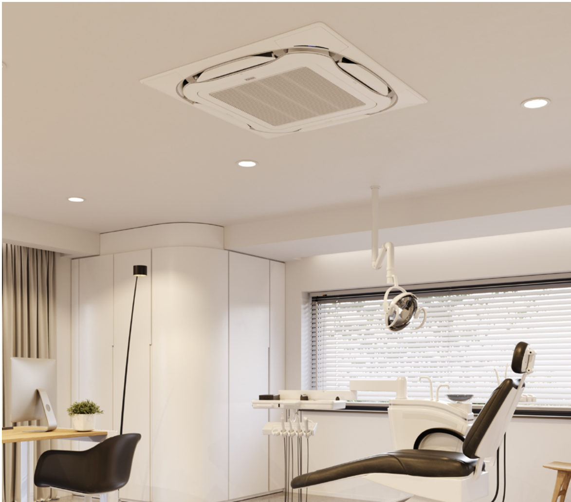
Round flow cassette, with UV streamer kit
